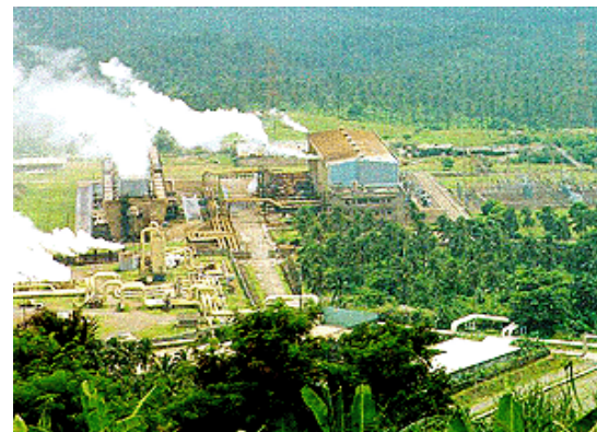
Makban Geothermal Power Plant Complex
