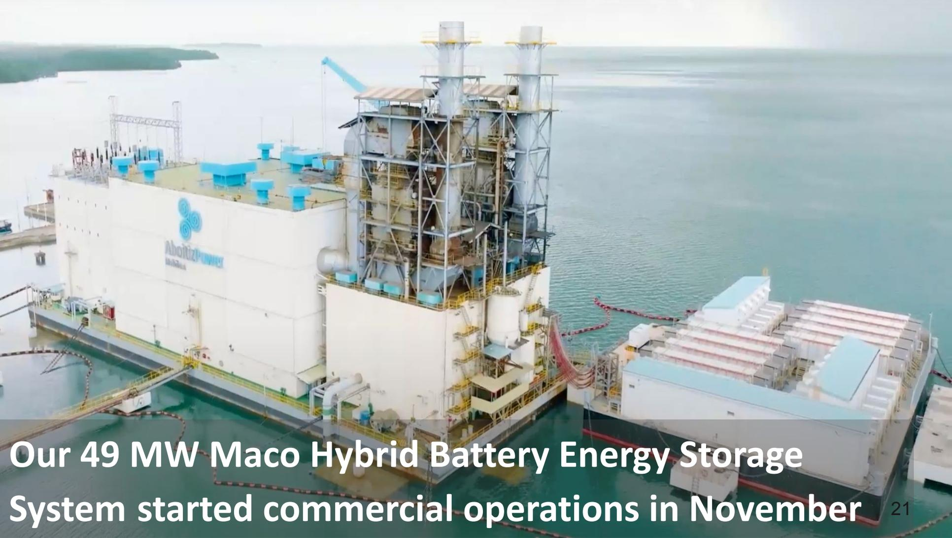
**Our 49 MW Maco Hybrid Battery Energy Storage System started commercial operations in November**
