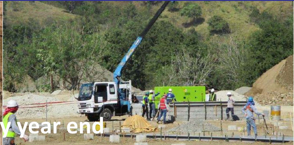
Temporary office pedestal installation
