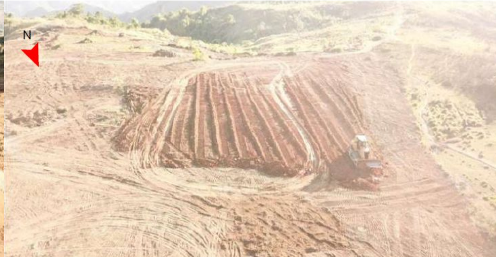
Grading works at the substation area
