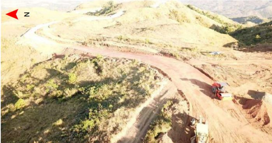
Road grading at PV plant site
