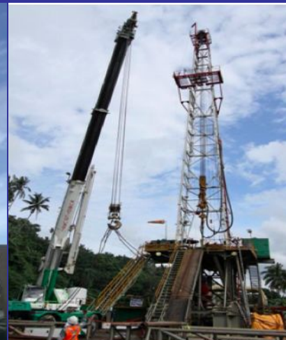
Tiwi Make-UP Well Drilling Rig in Operation
