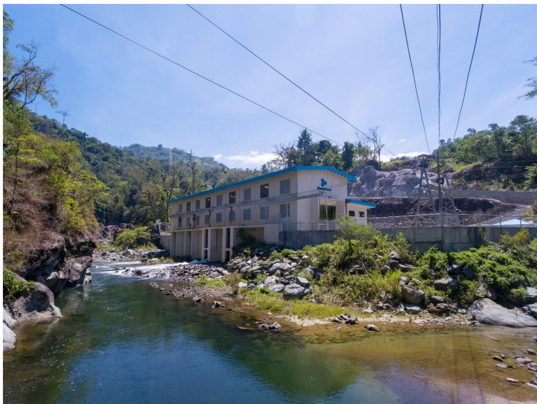
Hedcor's Manolo Fortich 1 Hydro Powerhouse
