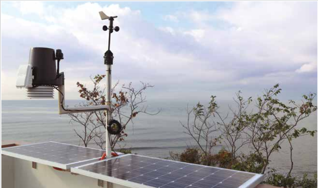
The automated weather station (AWS) is a stand-alone device that can accurately record temperature, pressure, humidity, solar radiation, wind, speed, and direction, as well as rainfall. The AWS complements local government efforts in generating variable weather knowledge and in enhancing their disaster preparedness and management plans.
