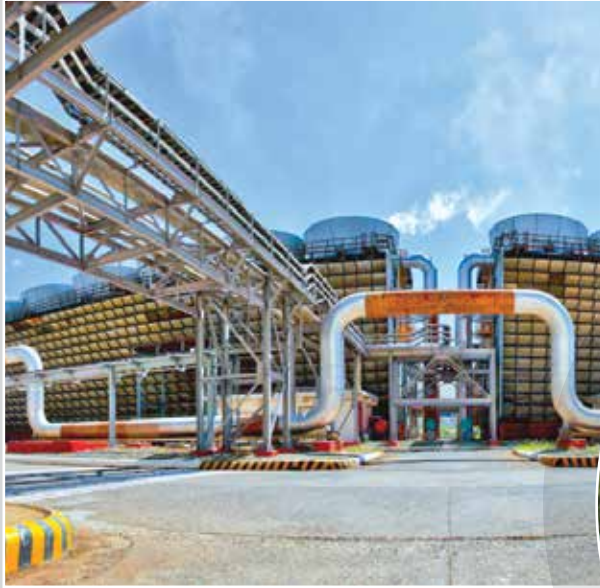
AP Renewables, Inc.'s geothermal power plants harness steam from the hot fluid recovered below the Earth's surface to generate energy, while the separated water is returned to the reservoir, helping to regenerate the steam source.
