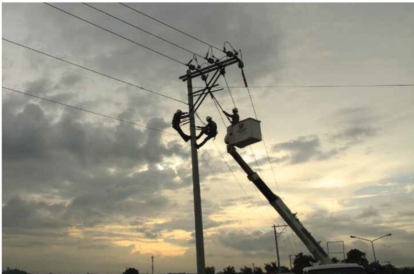
Davao Light linemen performing routine maintenance work
