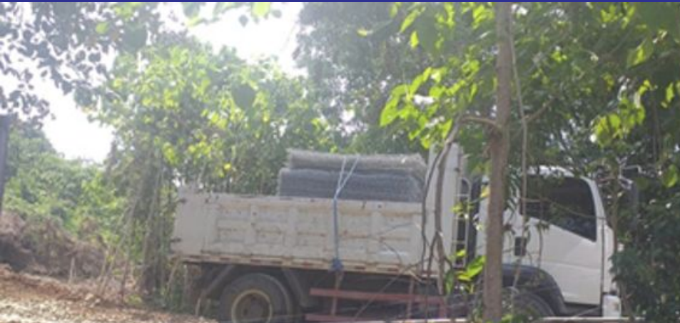
Delivery of slope protection materials
