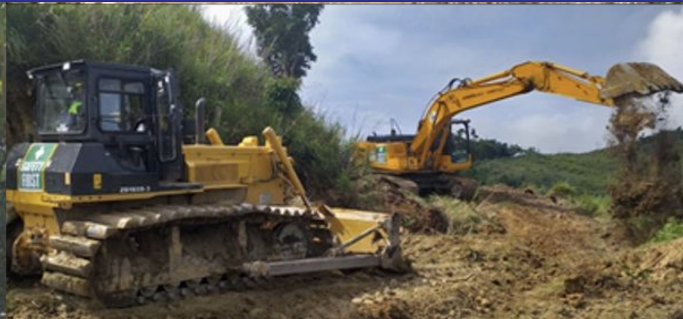
Widening along curves for accessibility of dumptruck
