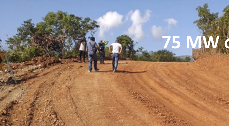
Joint inspection of excavation limits
