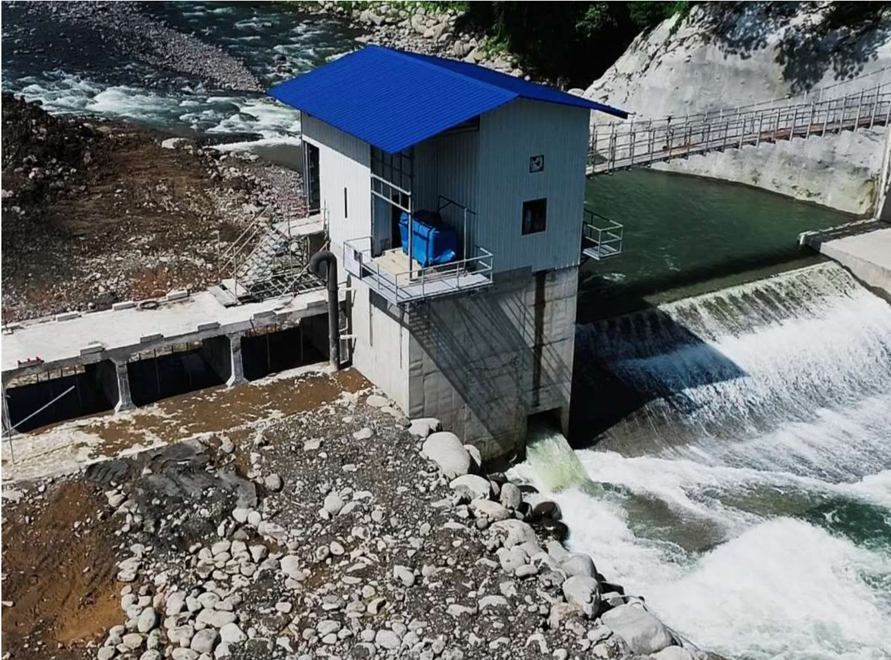
THE SHAPE OF WATER. Apo Agua has completed the construction of its run-off type intake weir across the Tamugan River, which will aid in managing the rate and volume of raw water diverted from the surface water source before it is conveyed to the water treatment plant.
