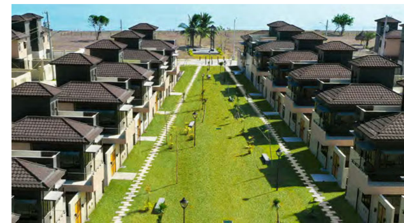
Apo Agua will shift Davao City's main water supply from groundwater wells to the more sustainably sourced surface water of Tamugan River.
