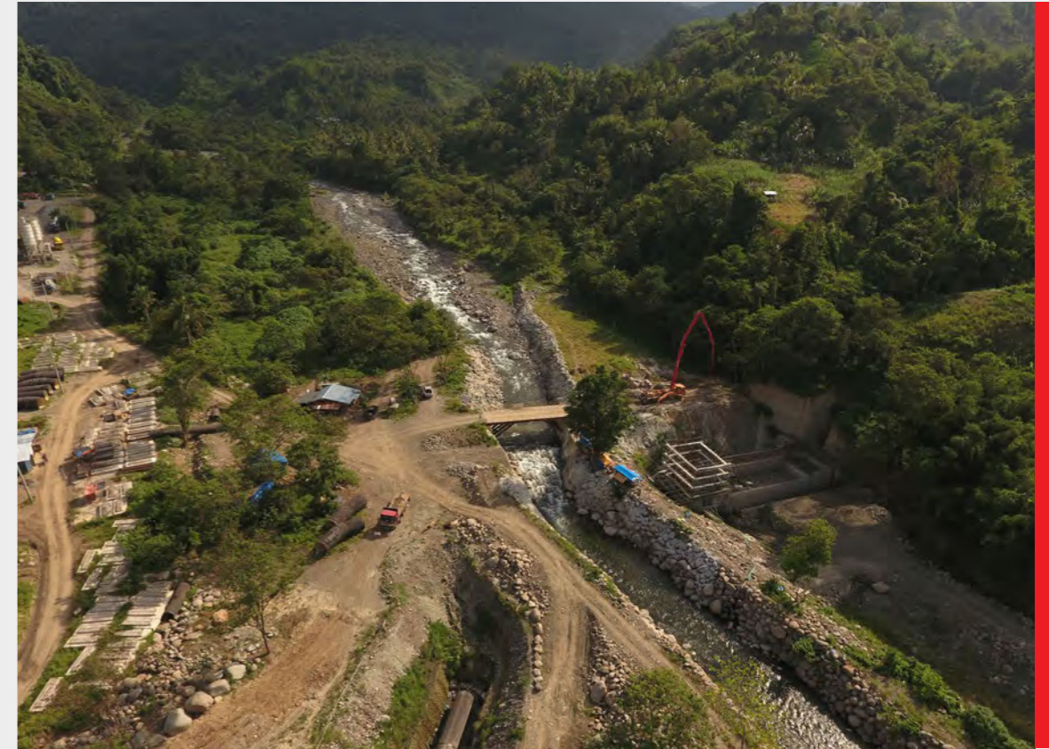
Construction continues for Apo Agua and JVACC’s bulk water supply project; above photo shows the intake weir being built at Barangay Tawantawan, Davao City
