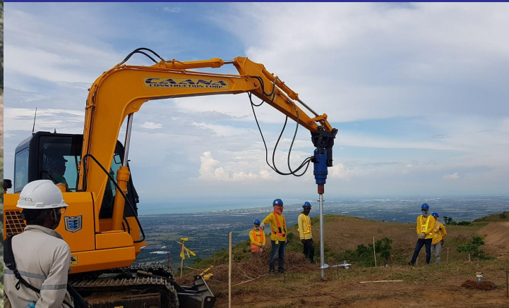
Screw Piling Works at PV Area
