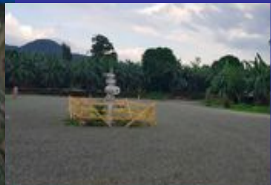
MGP roads and rig staging areas ready
