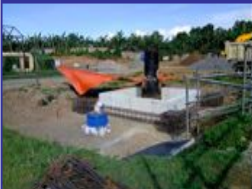
MGP production well pads ready for drilling
