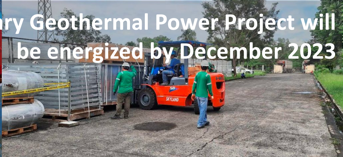
AIR COOLED CONDENSER COMPONENTS DELIVERY
